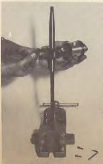
Fastening the connecting rod to the crankshaft.
