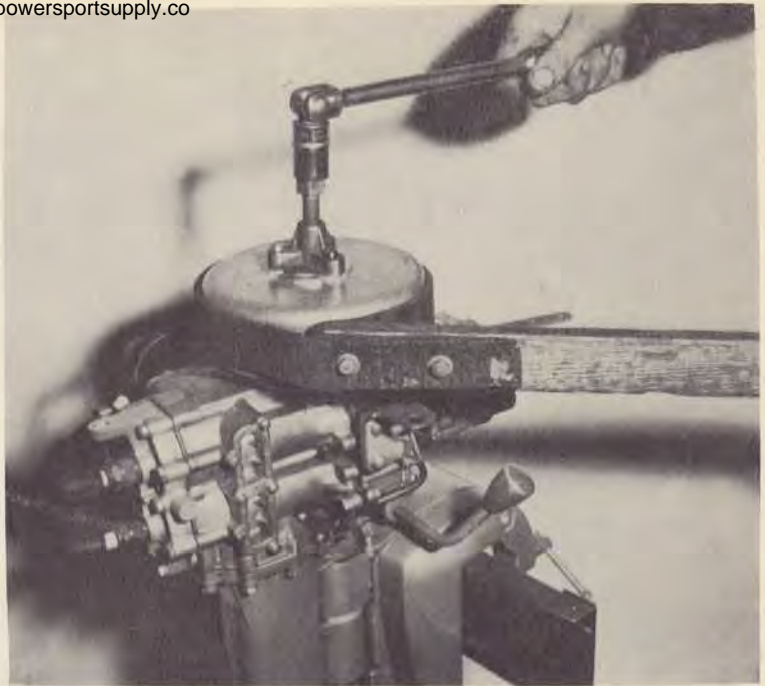
Using flywheel puller and home made holder.
