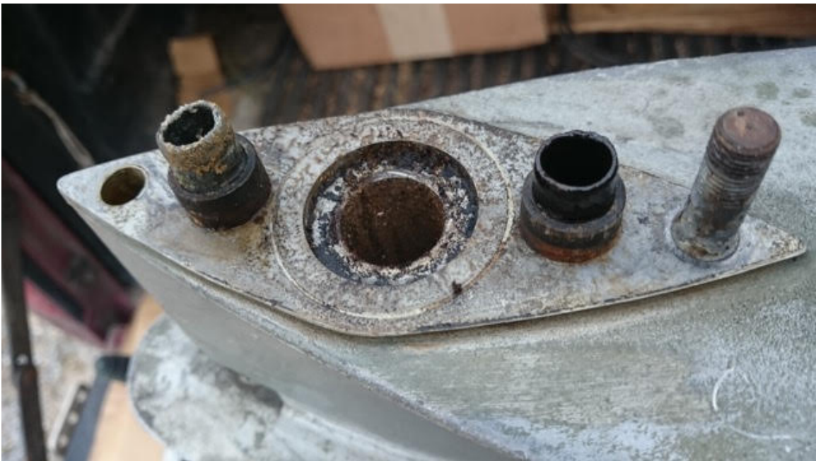
View of the supply hole from the water pump (right hole) and the blind hole (left hole) that the Y pipe fits into. (See picture below)
