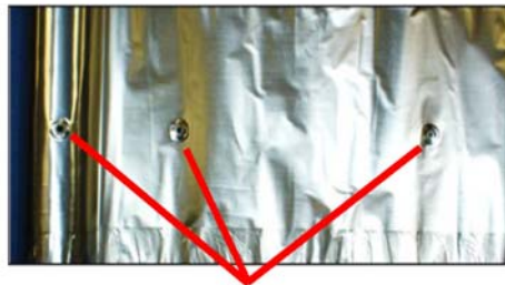
Pinholes / arcing through the film insulation. (75X magnification).
