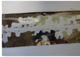
Plate failure due to corona discharge (high voltage + air gaps in the windings)
